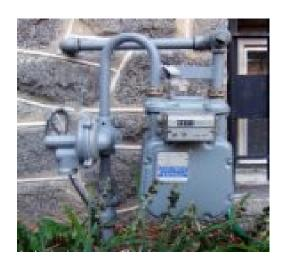
It's important to know exactly where your gas meter is located and how to shut it off in case of emergencies. All you need is a 12" adjustable wrench!
