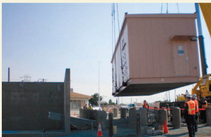
Prefabricated MCC being lowered into position
