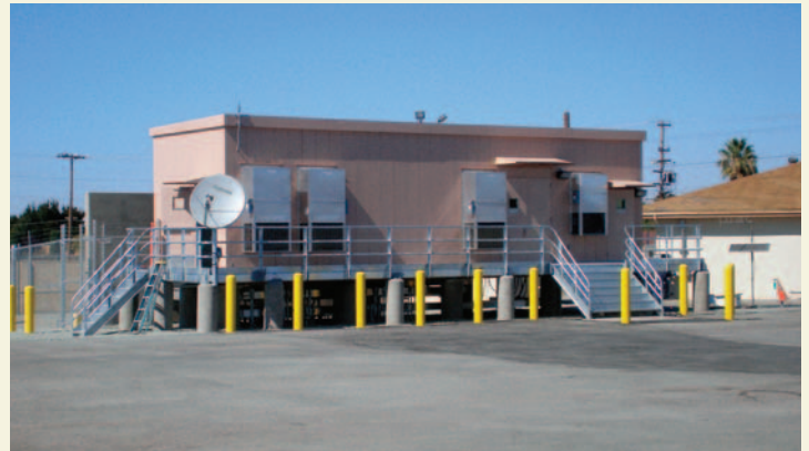
Completed MCC building
